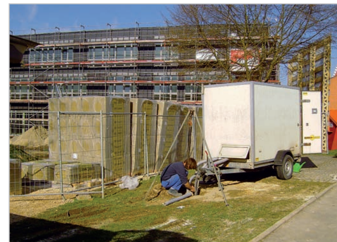
Geothermal Response Test
